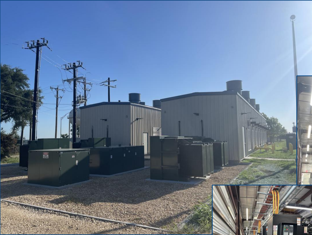
16 Generac SG625 units Utility connected, remotely dispatched RPower Turnkey Design and Build
