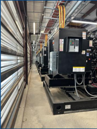
16 Generac SG625 units Utility connected, remotely dispatched RPower Turnkey Design and Build
